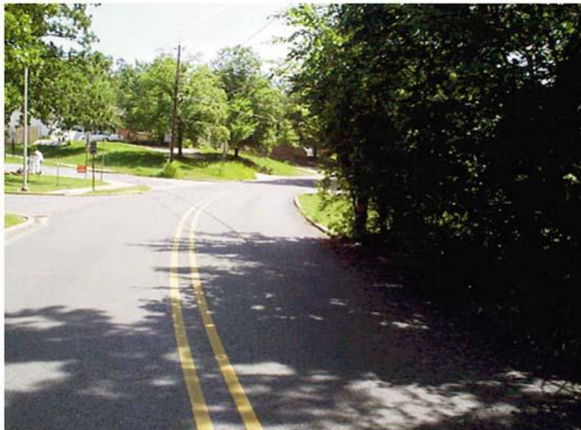
Figure 2. An example of lack of attention to plant growth along the street
