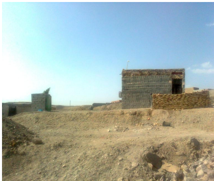
Figure 3: An example of illegal construction in Iranshahr
